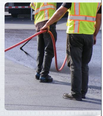
Remove all broken asphaltic concrete and prime and patch area with new asphaltic concrete based on manufacturer's recommendations. Wash, sweep, blow, or vacuum surface to assure a clean bondable surface.
